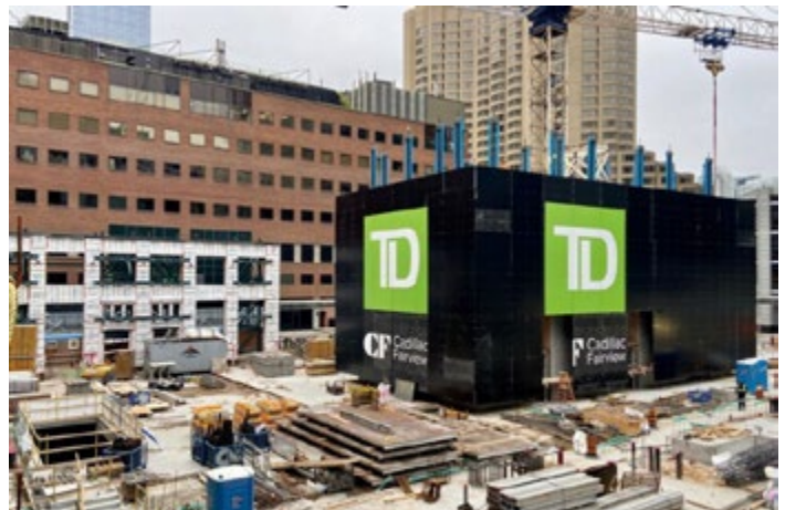
165 Front Street. Being built by PCL is a Cadillac Fairview property that will provide a new location for TD Bank
