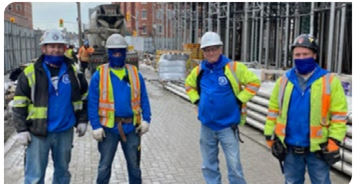
Local 1030 members on site at Atriacon Developments in Oshawa. On Bond St. and Mary St. High rise building Project
