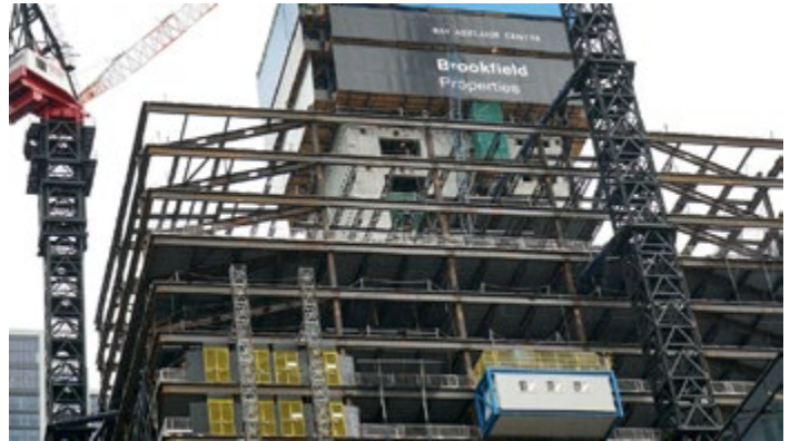
DON PROCTER – At Bay and Adelaide Streets in downtown Toronto the 32-storey Scotiabank North Tower is rising with a hydraulic climbing system made by Doka. It is the second time the Doka climber, which consists of three integrated systems, has been used in Toronto by Structform.
